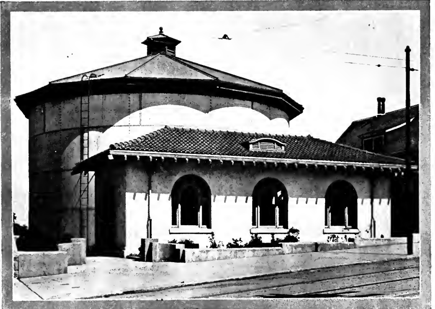
ASHBURY HEIGHTS PUMPING STATION
